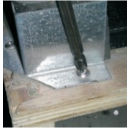
Image 2 Removing bracket from cabinet
